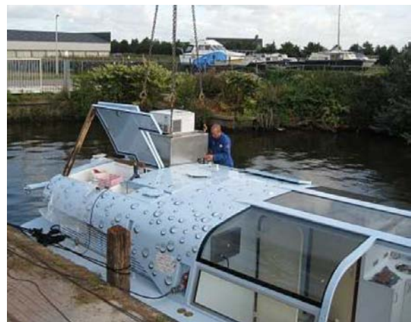
Figure A.5: Installation of Fuel Cell Module at Nemo H2
