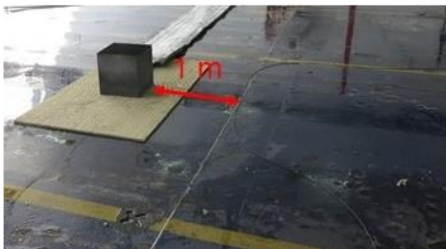
Figure 22. Position of the fibre optic cable on the floor.
