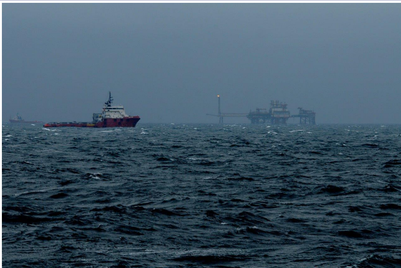
GSP Orion conducting pollution response exercise in the vicinity of the Central Production Platform
