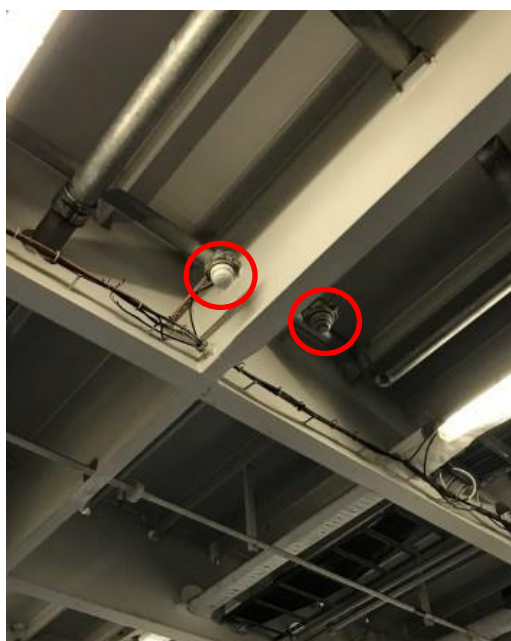
Figure 6: Point detectors locations (new and old detectors)
