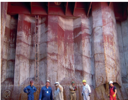
EMSA will look to streamline the inspection task and thereby enhance its effectiveness.
