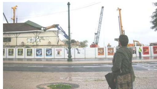
Work began in mid October on the permanent EMSA headquarters at Cais do Sodré in the historic centre of Lisbon. The initial works involve the construction of purpose-built wells for lowering the ground water in the area, the destruction of an old warehouse (above) and the preparation of the ground for the next phases of construction.
