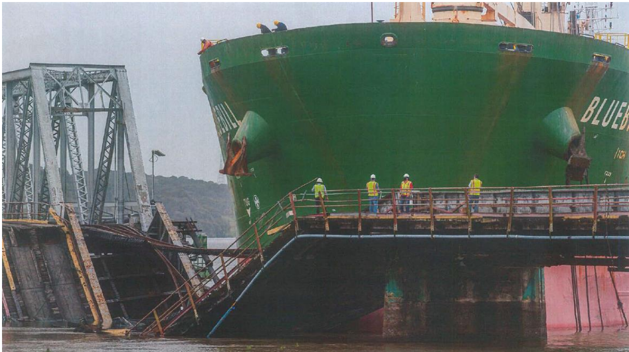
Contact of MV Bluebill with the Old Gaboa Railway Bridge in Panama Canal on 23/06/2020, following a loss of control / direction power.
